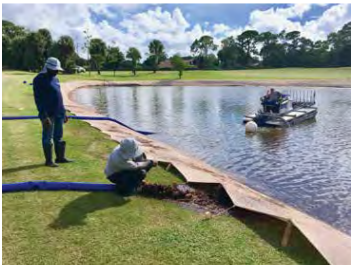
Shallow pond sediment is pumped with our amphibious work boat directly into the SOX containment system to restore the shoreline.
